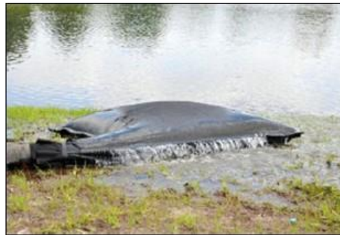
Plate 2 Silt bag with water being pumped through
